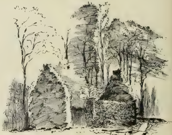
FIG. 1443.—Auchterarder Church. View from South-West.
